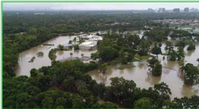
Overview of Flood Water at Lakeside CC
